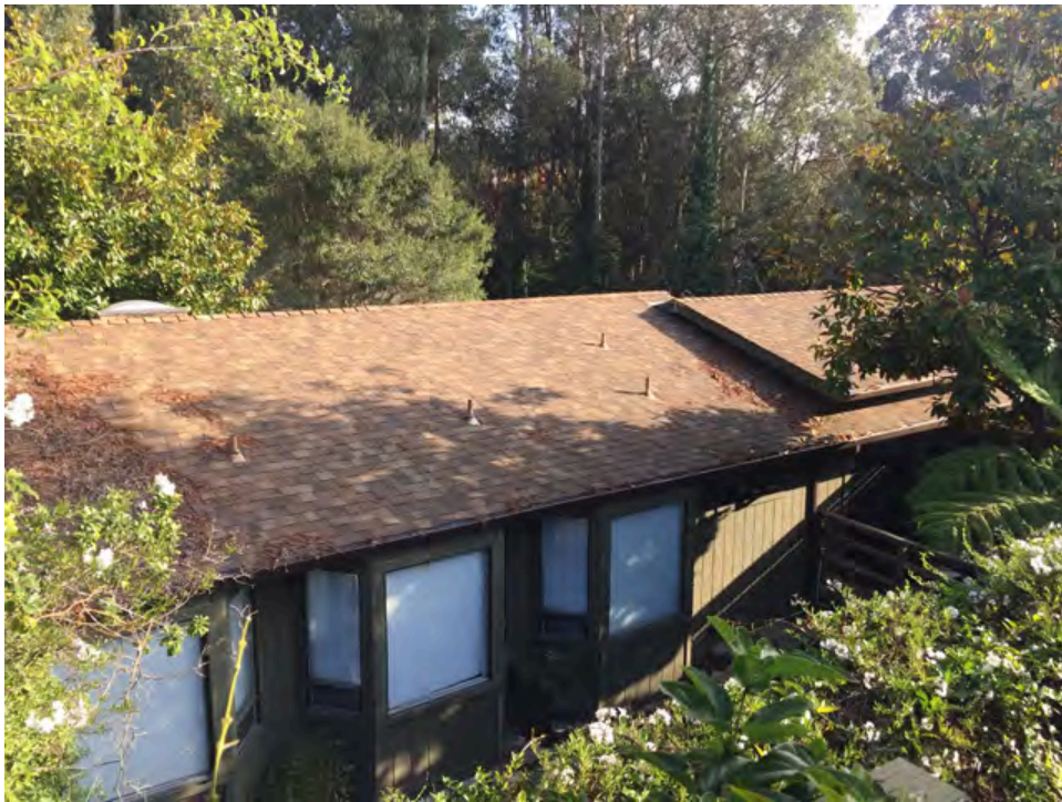
4. View of commercial-only building
