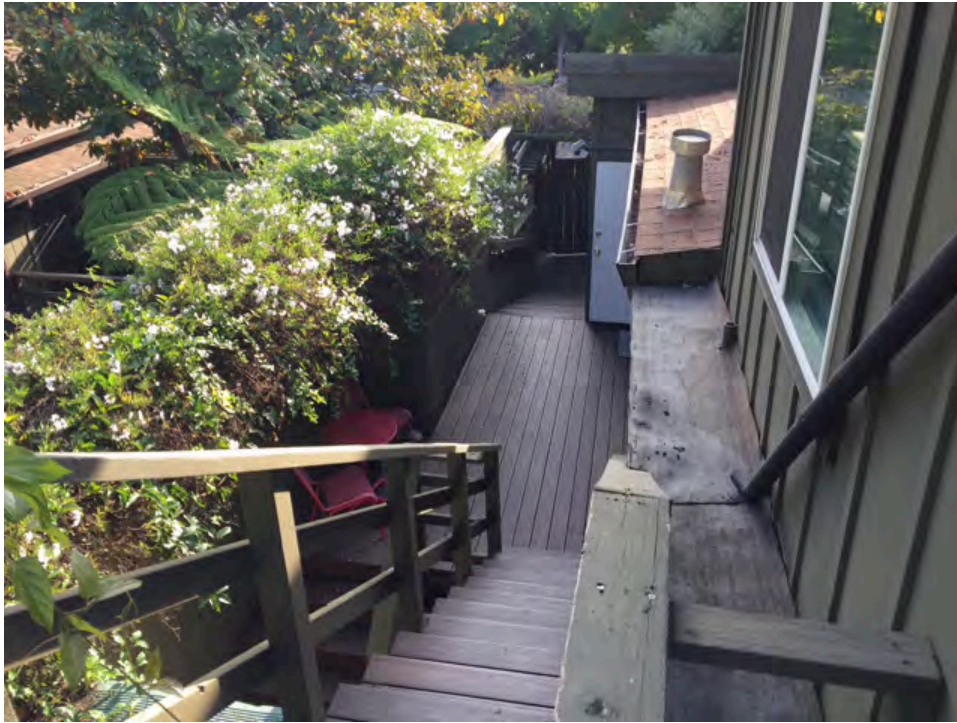
7. Stair access to residential unit
